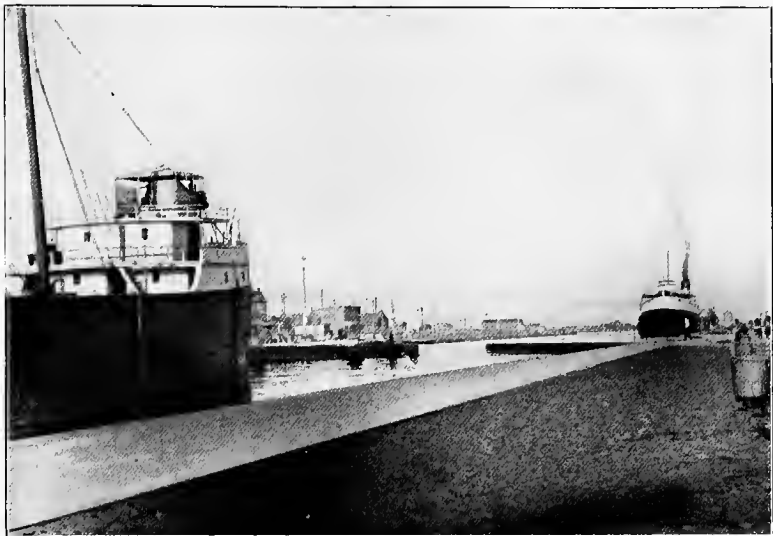
IN THE UPPER WEITZEL LOCK, ST. MARY'S RIVER CANAL
